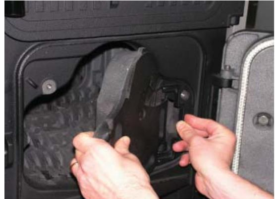
Fig. 14 Remove the grille
