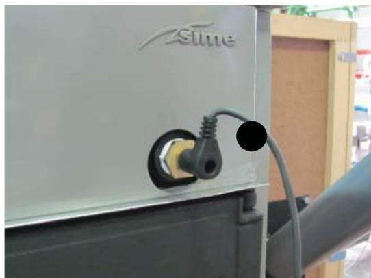
Fig. 34 Safety thermostat connector
